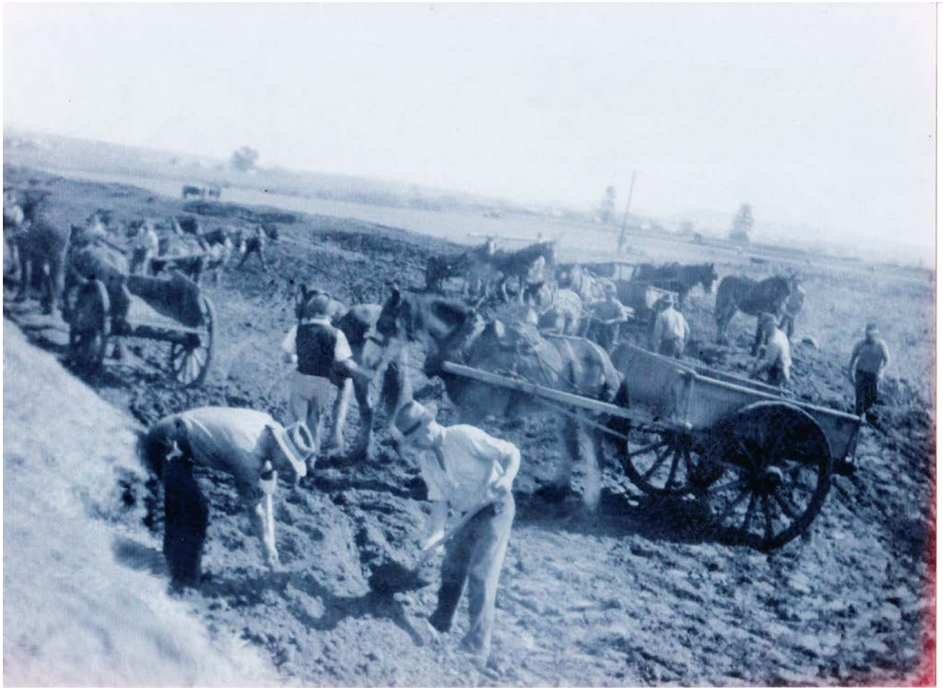
Figure 3: Fourteen men, thirteen horses and six drays working on a Bolwarra embankment in 1950: in the foreground are Bob Hungerford (with pipe) and Les Mead
