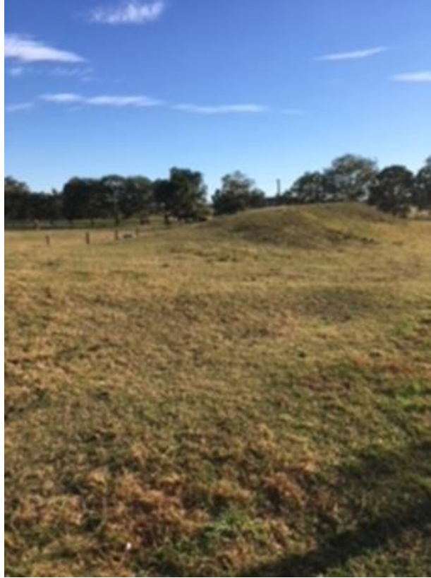
Figure 2: A nineteenth century levee on the Pig Run meander, next to Glenarvon Road
