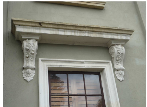
4. The 1860's masonry work is superb. Only minor changes are apparent.
